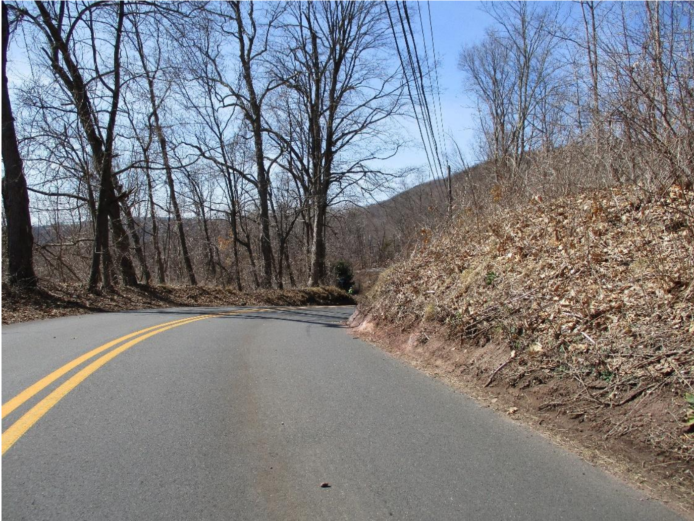
Westbound Mount Carmel approaching Outer Ridge
